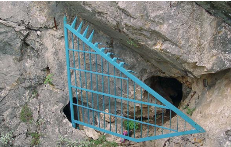
This gate restricts the number of bats that can fly through it at any time
