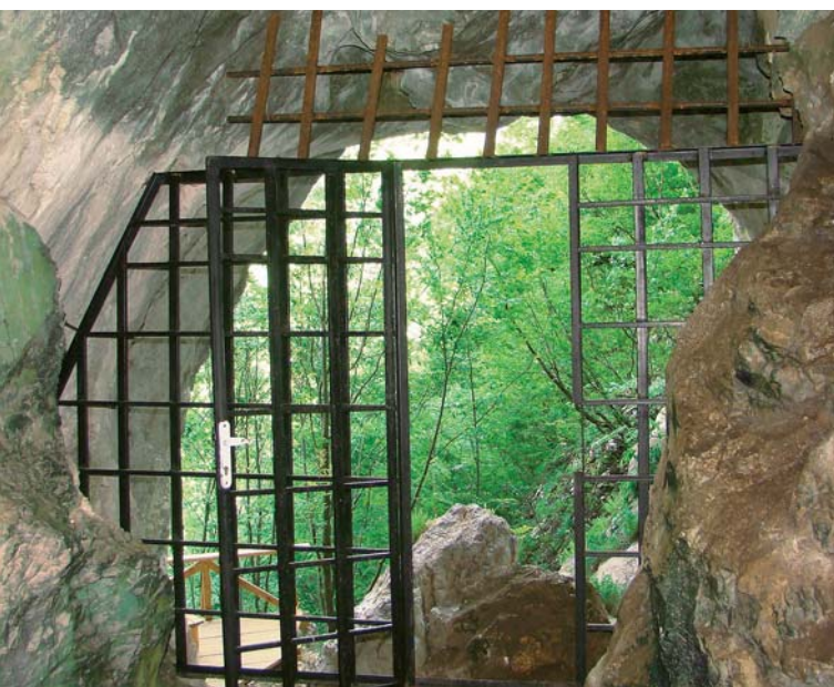
Bad gate: small square holes which hinder the free flight of bats
