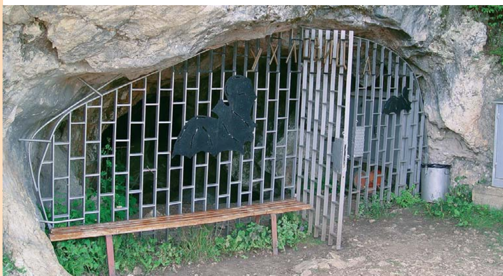
Though a bat silhouette is hanging at the entrance of «Uhlovitsa» cave in the Western Rhodopes Mt., design of the gate does not allow enough room for bats to fly through
